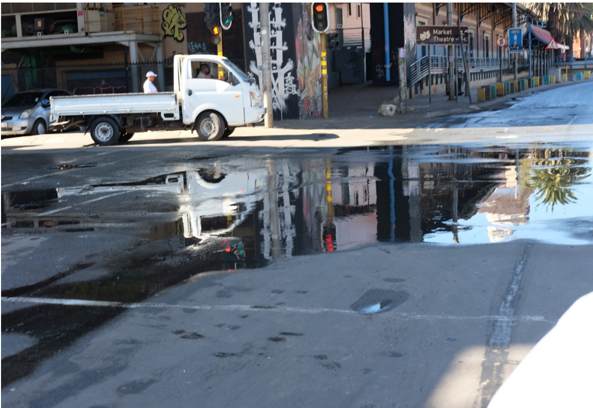
Water leaks in central Johannesburg. The city's fragmented governance structure has heavily affected the level of expertise and quality of service delivery. Photo supplied
